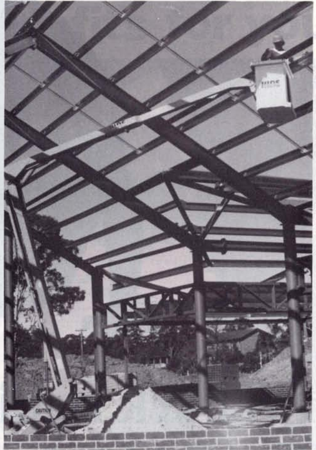
A 12 metre trailer lift, from Kennards Hire, in use on the new church being built at Austral.
